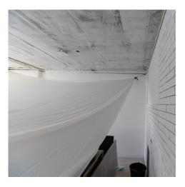
• Begin at one corner and gradually insert the edge of the film into the track.
