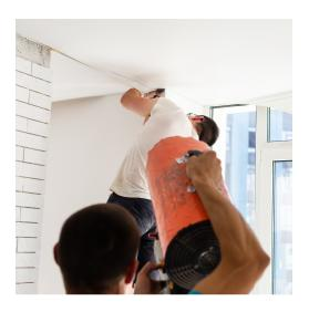
• Ensure the material is evenly tensioned and securely fixed into the track.
